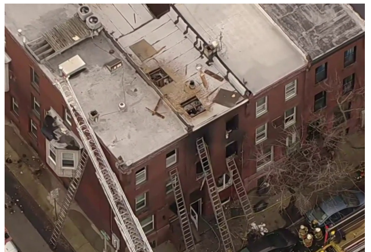
Philadelphia, PA January 5, 2022 A three-story duplex in Philadelphia caught fire, trapping 12 victims in the city's deadliest fire in more than a century. Four smoke detectors inside the row house were not working, according to fire officials.
